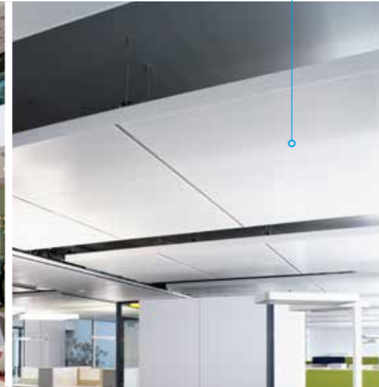
Ceiling rafts (p.22)
